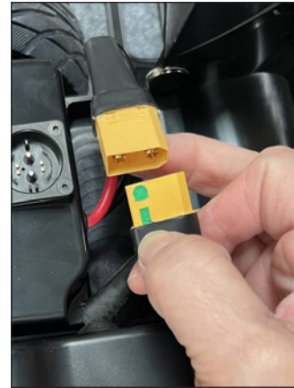
Figure N: Battery disconnected.
